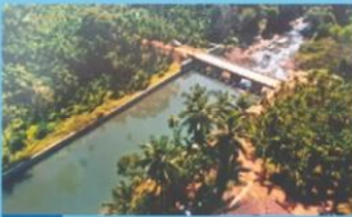
Construction of KINDI Dam at Belthangadi Taluk, Southcanara District
